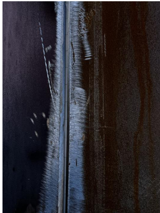
3229 – Mater Butt Joint ready for welding
