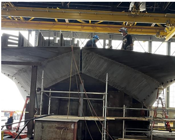
3004 – Module 1 with most of hull plating in place
