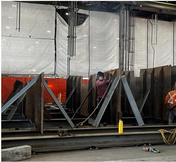
3039 – The Falsework Gig for Module 5
