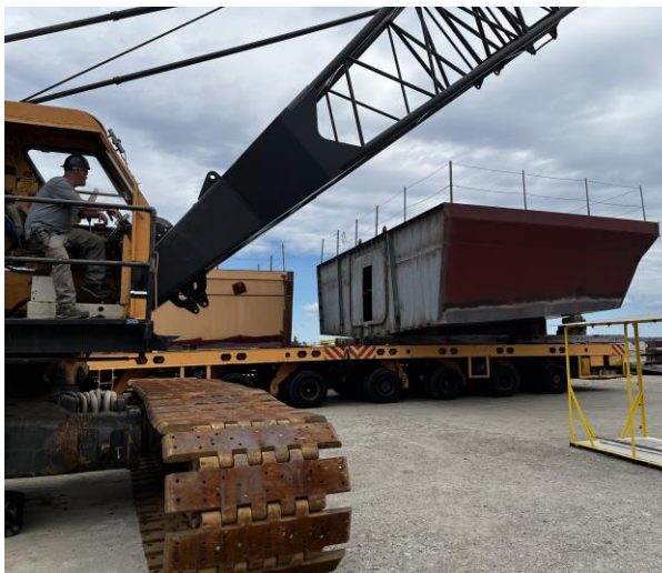
3099 – Module 2 heading for the Erection Runway
