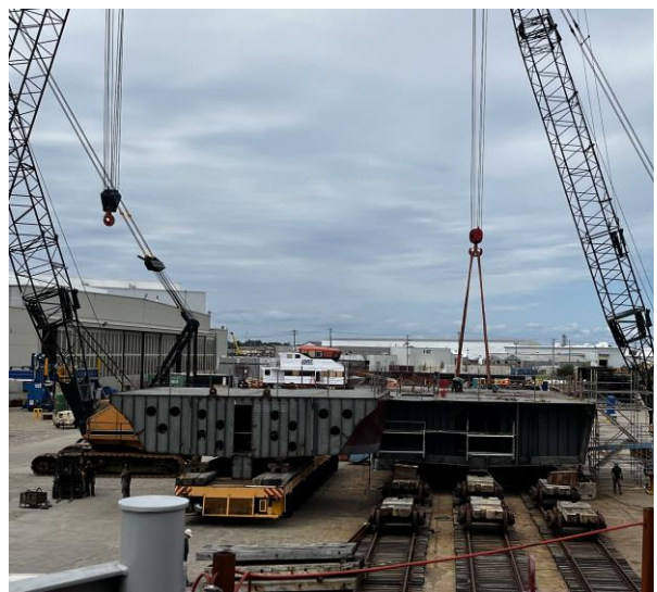
3100 – Module 2 being lifted into place on the Runway
