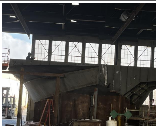
2986 – Module 1 with Bulkheads being fitted
