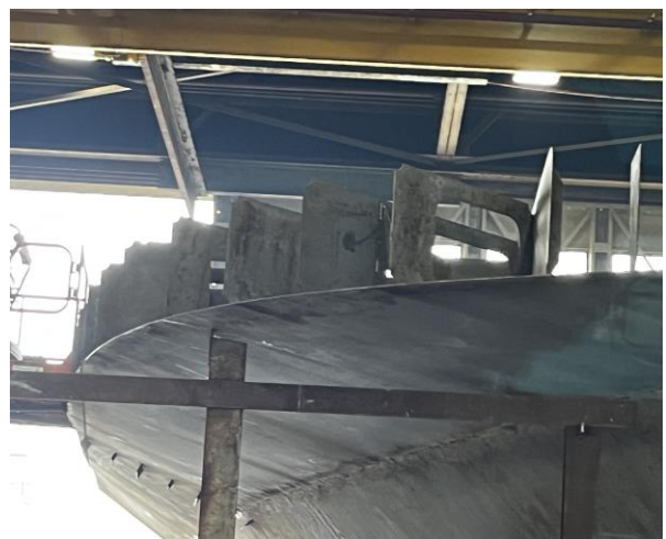
3005 – Module 1 Guard framing being installed
