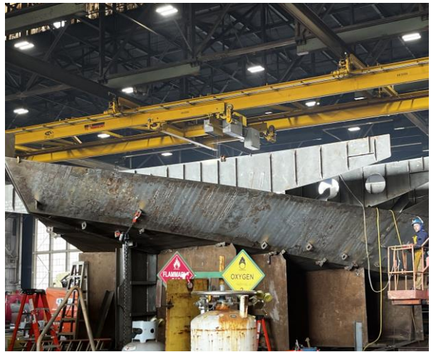
3152 - Module 5 having side shell hull plating installed
