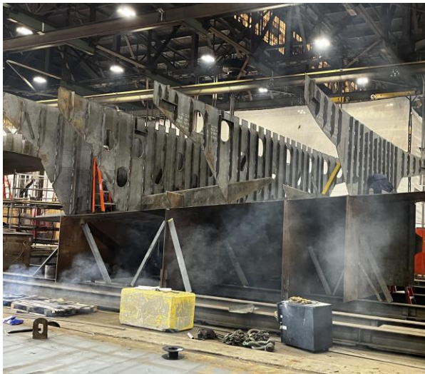
3120 – Module 5 Transverse Bulkheads in-place
