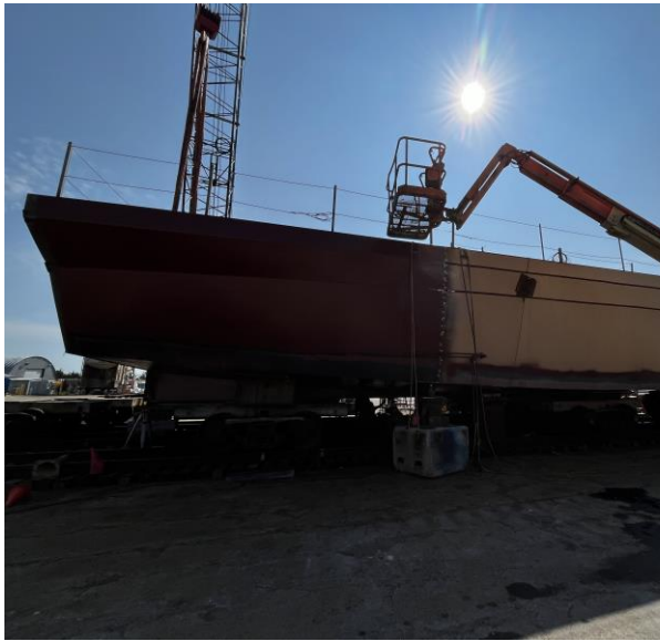
3078 – Preparing the Master Butt (seam) between modules 3 & 4
