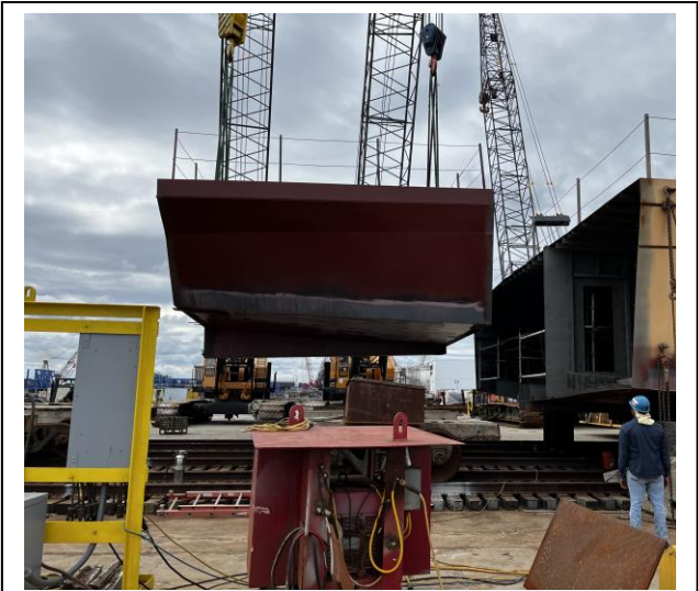
3103 - Lifting Module 2 into place on the Runway
