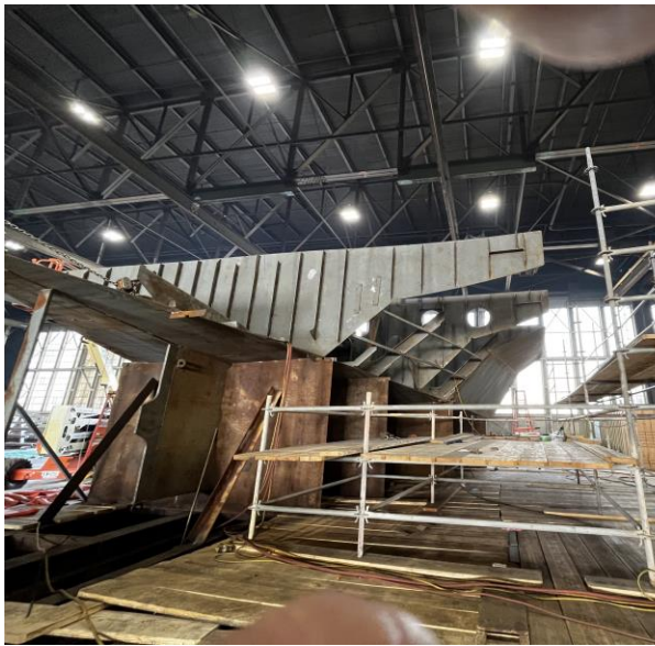
2988 – Module 1, Port side with side hull plating just getting started
