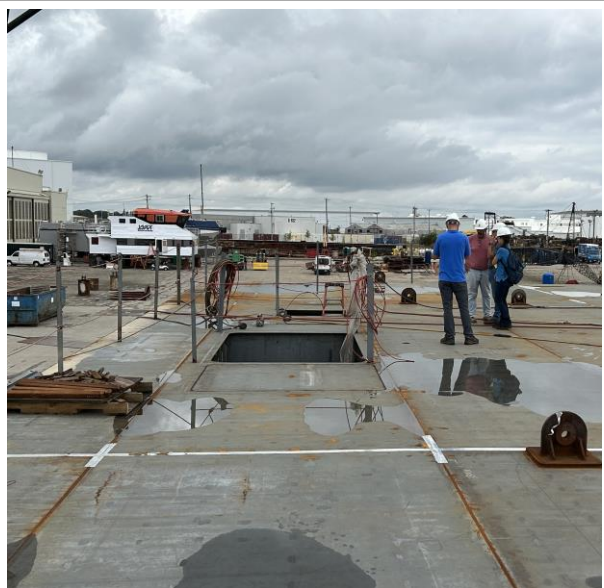
2376 – On the deck of modules 2, 3 & 4 with elevator pit next to people
