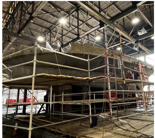
3058 - Module 1 Guard plating being installed – Port Side
