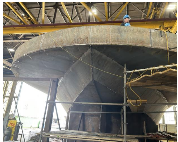
2370 – View of Module 1 from below the bow
