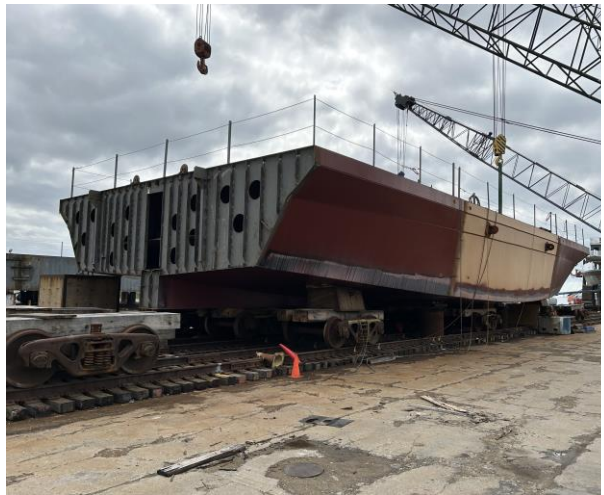
2371 – Modules 2, 3 & 4 aligned on Erection Runway
