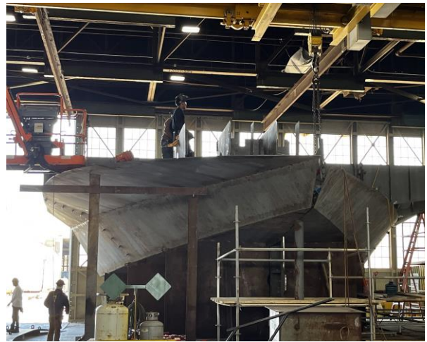
2997 – Module 1 with more Port side plating being installed
