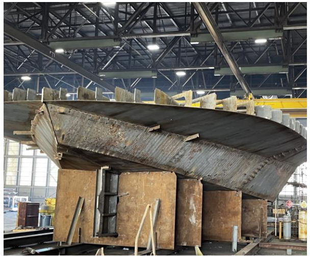
3232 - Module 5 with Guard framing in place
