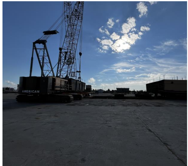
3041 – Preparing to lift Module 4 onto the Erection Runway
