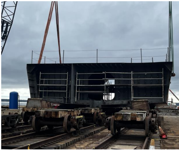
3032 – Module 3 being lifted onto the Erection Runway
