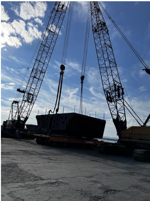
3040 - Module 3 being lifted onto the Erection Runway
