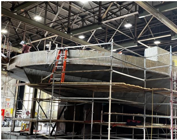
3165 – Module 1 with weights holding deck plating flat
