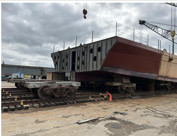
2372 - Modules 2, 3 & 4 aligned on Erection Runway
