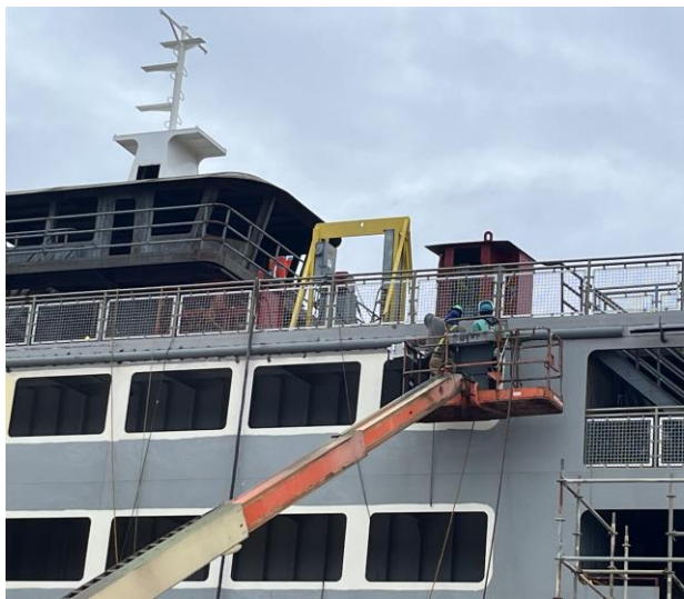
5106 – Installing pipe guard at 02 deck level
