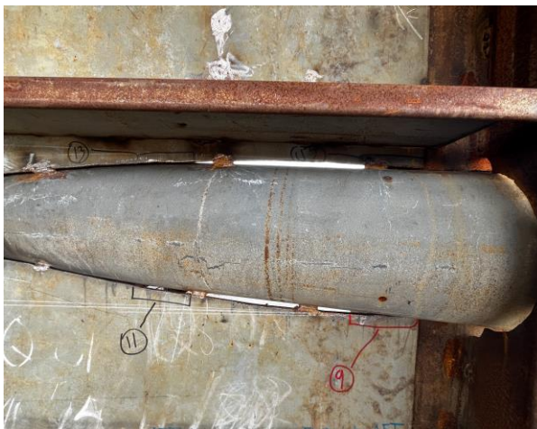
4913 – Stern Tube Tack Welded and Marked to control movement
