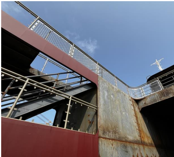
4892 – 02 Deck Railing as seen from Main Deck
