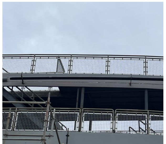
5107 - Installing pipe guard at 02 deck level
