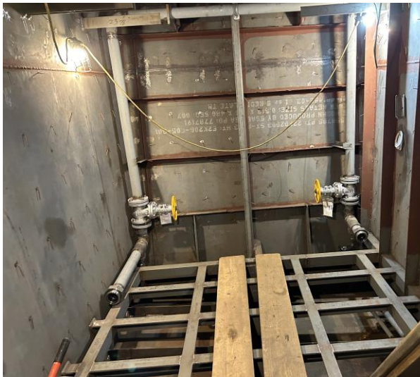
2595 – Battery Foundation Framing with Off-Gassing Piping
