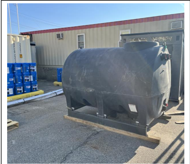
5017 – Sanitary Sewer Tank
