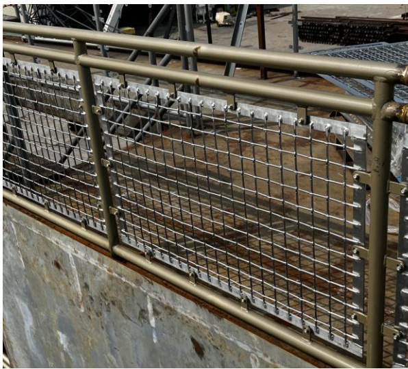
4890 – Screen Section Connections
