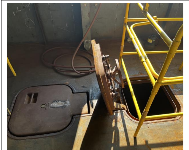
4873 – Hatch from Engine Room
