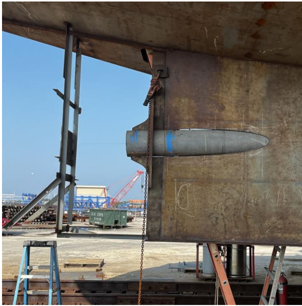
4881 – Aligning Stern Tube Before Welding
