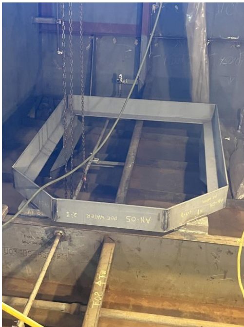
5041 – Support Frame for Potable Water Tank
