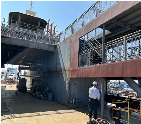
2587 – Handrails coming together throughout the vessel
