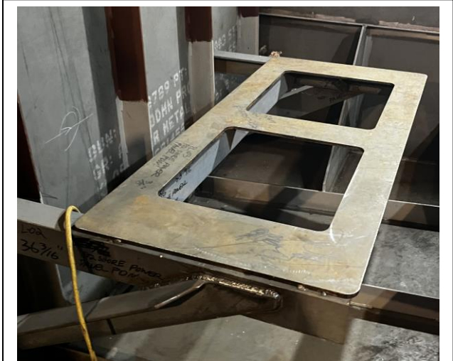
4878 – Foundation Frame for Shore Power Panel in Switchboard Room
