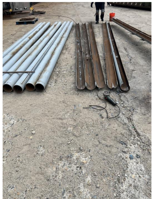
5103 – Guard Piping split in half for installation
