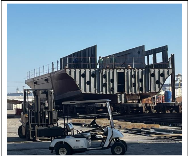
3284 – 1 st Module 7 Bulkhead for Main Deck Starboard Cabin
