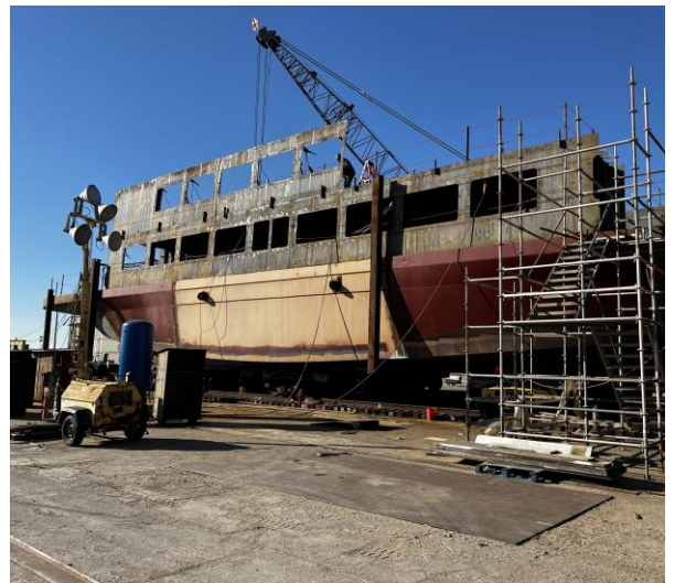
3461 – Setting Module 10 Bulkhead (01 Deck Cabin) on Port Side
