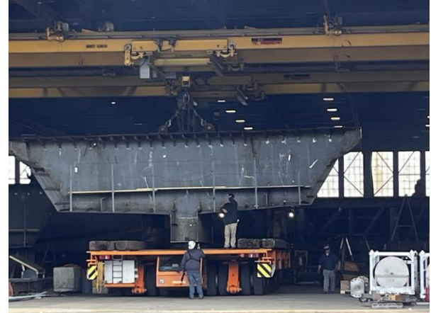
3350 - Module 1 Lifted and Almost Set on the Trailer
