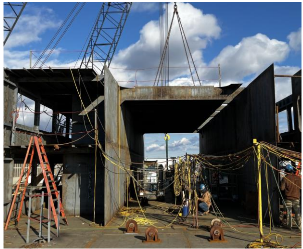
3505 - Placing 02 Deck Plating Over the Vehicle Alleyway
