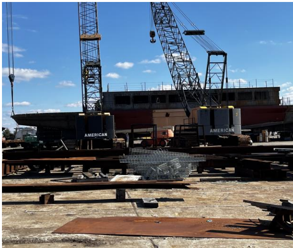
3442 – Module 5 Being Aligned with the Other Modules
