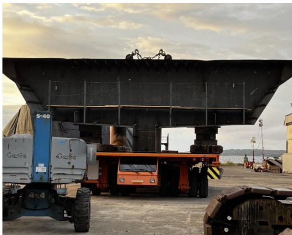
3352 – Module 1 Heading Towards the Assembly Area (Erection Yard)
