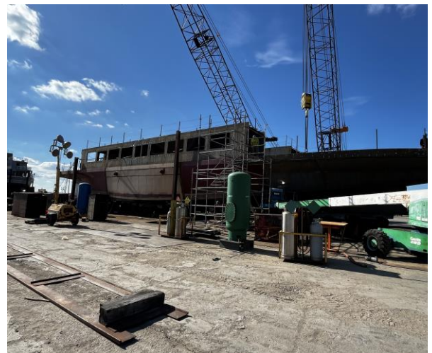
3445 - Module 5 Being Lifted onto the Blocking in the Assembly Area
