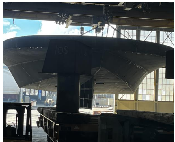
3346 - Module 1 Lifted and Ready to be Loaded on Trailer, Moving Trailer Under the Module
