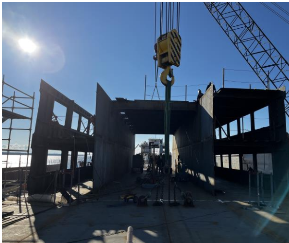
3502 – Placing 02 Deck Plating Over the Vehicle Alleyway
