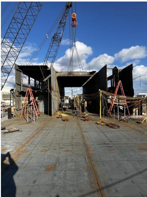
3506 - Placing 02 Deck Plating Over the Vehicle Alleyway
