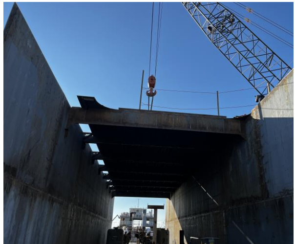
3503 - Placing 02 Deck Plating Over the Vehicle Alleyway
