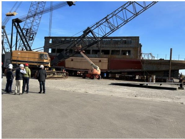
2419 – FTA Site Visit, Looking at Starboard Side of Vessel
