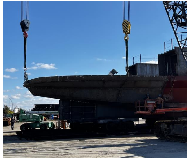
3443 – Module 5 Being Lifted onto the Blocking in the Assembly Area
