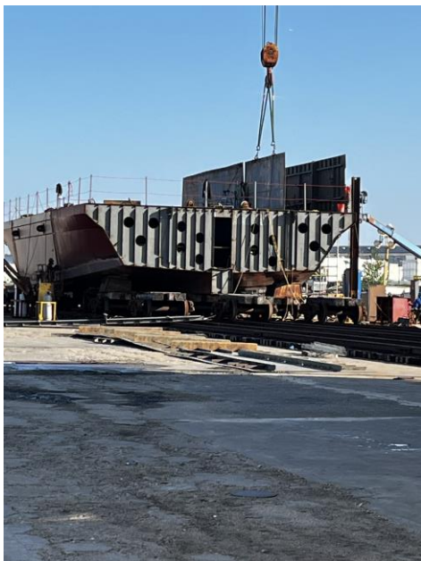
3277- Setting Module 7 Bulkheads (Main Deck Cabin – Port Side)
