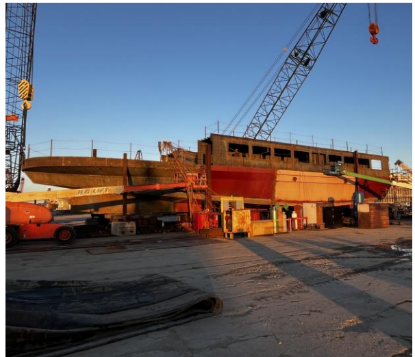
3426 - Port Side View of Vessel with Module 1 in Place
