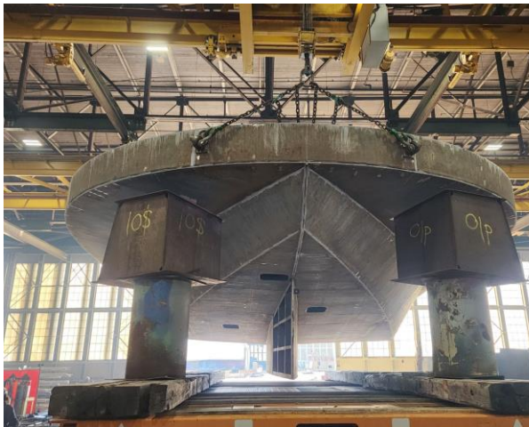
9556 – Module 1 (Bow-Peaks End) Ready to be Moved to Assembly Area.
