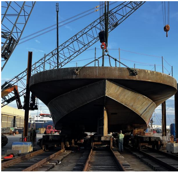
3381 – Module 1 Setting on the Erection Blocking
