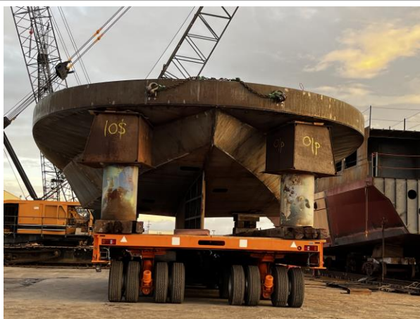
3354 – Prepping Module 1 for Lifting and Aligning with Modules 2, 3 & 4
