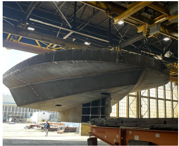
3344 - Module 1 Lifted and Ready to be Loaded on Trailer, Starting to Move Trailer Under the Module
