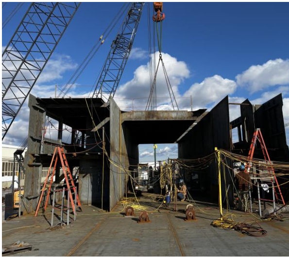
3504 - Placing 02 Deck Plating Over the Vehicle Alleyway
