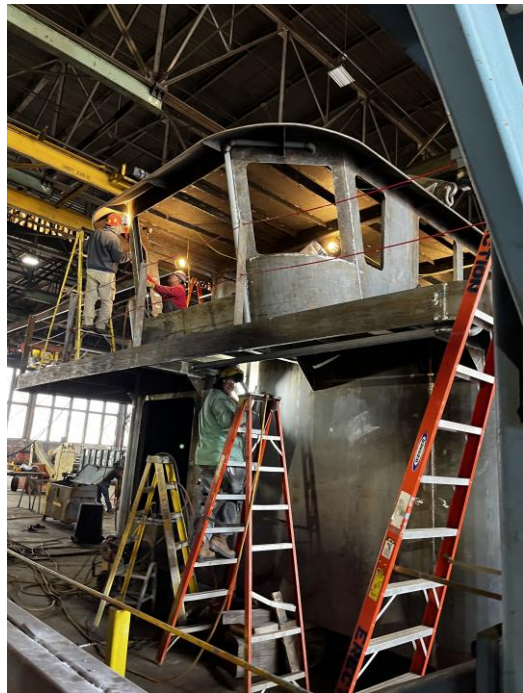
4292 – Work Being Done on Pilot House
