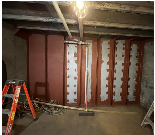
4297 – First Coat of Paint in 02 Deck Cabin
