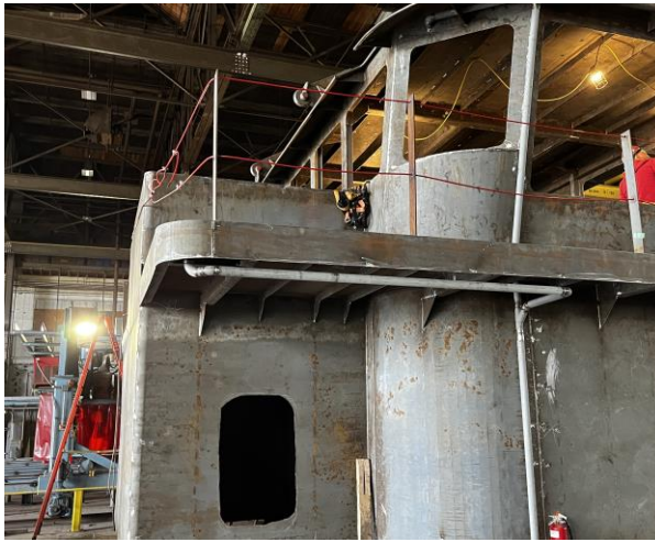
4290 – Drain Piping Around Pilot House
