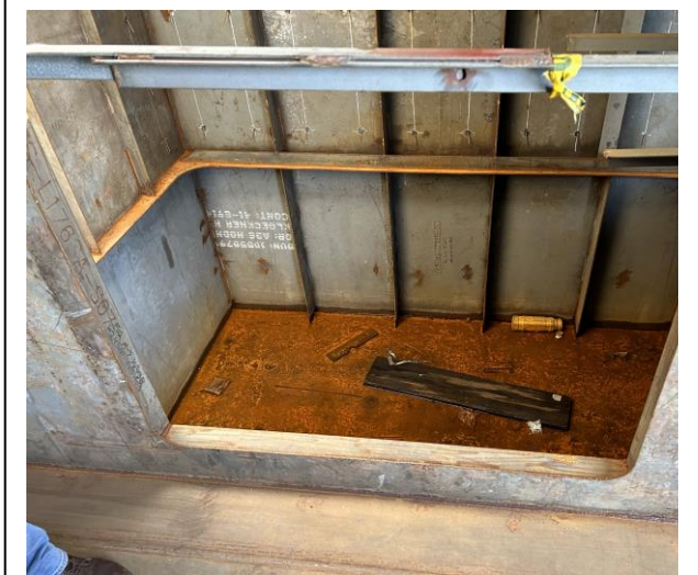
2519 – Elevator Pit at Main Deck
