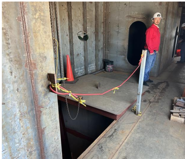
2517 – Access Opening for Equipment Drop to Engine Room
