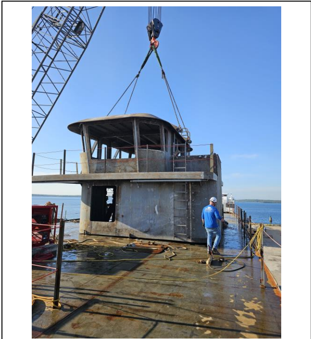
71903 – Pilot House Set in Position on 02 Deck
