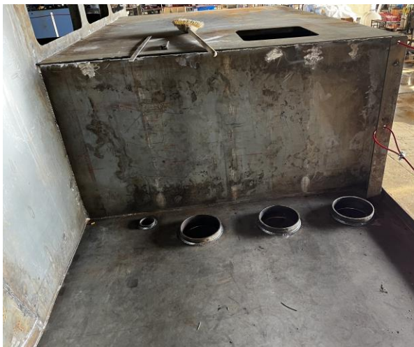
4379 – Exhaust Piping Penetrations at Pilot House
