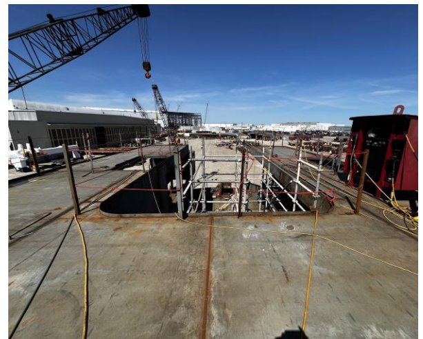
4236 – View Aft to Stern from 02 Deck
