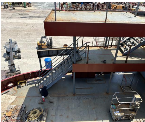
2531 – Port Stern Stairs as Seen from 02 Deck
