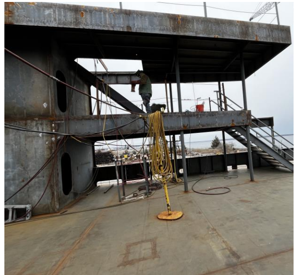
4161 – Working Handrails on 01 to 02 deck Stairs on Port Bow
