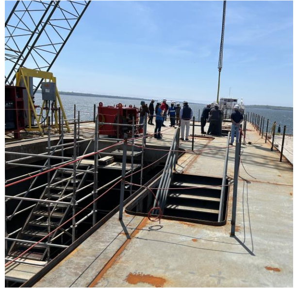
2530 – Looking Across 02 Deck Before Pilot House was Set
