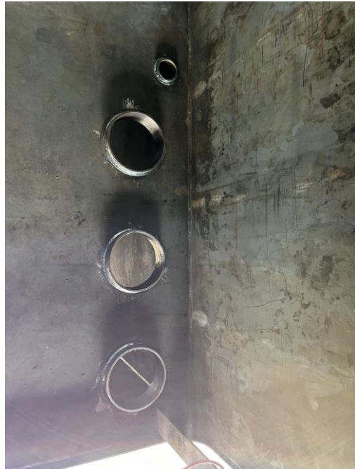
4378 – Exhaust Piping Penetrations at Pilot House
