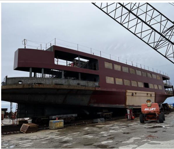
4293 – First Coat of Paint on Starboard Side
