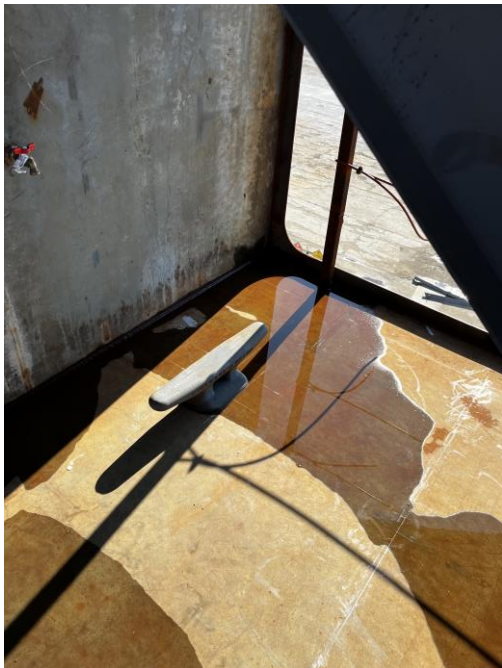
4569 – Cleat Install Location
