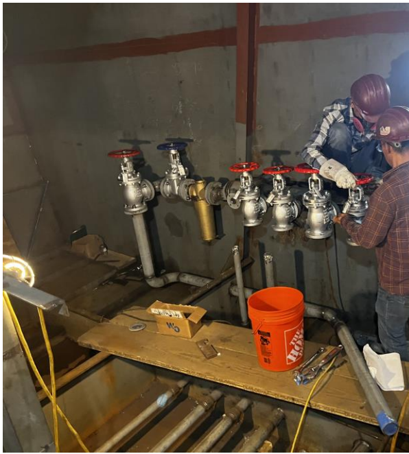
4750 – Valves Being Installed on Manifold
