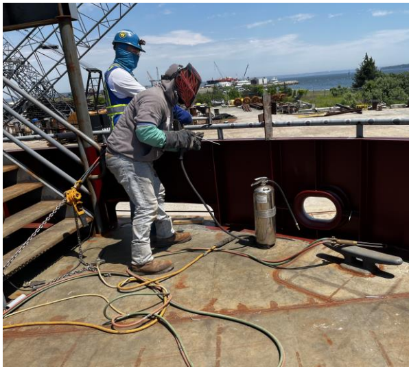
4504 – Installing Rail on Top of Bulwark
