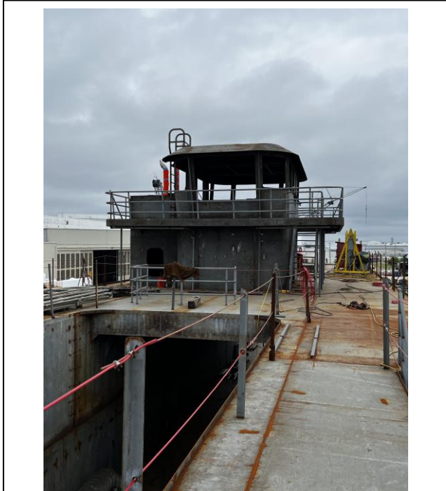
4657 – Handrail Installed Around Pilot House
