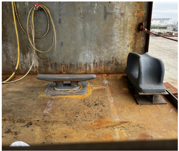
4659 – Cleat Installed & Line Chock Set & Tacked
