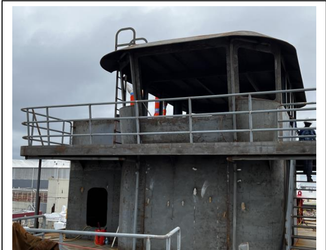
4655 – Handrail Installed Around Pilot House
