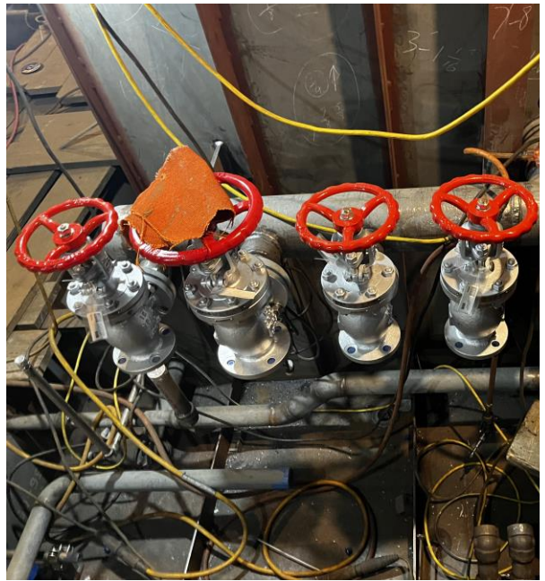
4751 – Valves Being Installed on Manifold
