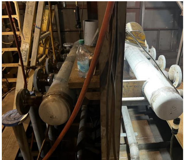
4720 – Piping Manifold Being Installed
