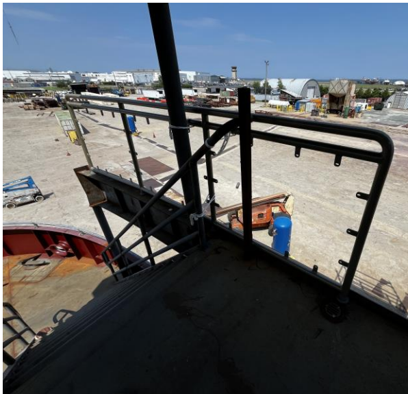
4721 - Pedestrian Handrail System being Installed
